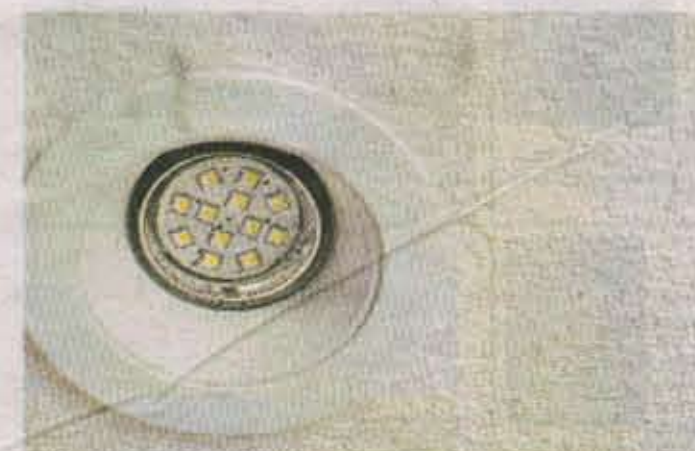
LED lights have replaced the kitchen's mundane fluorescent tubes. The LEDs last longer, too.
